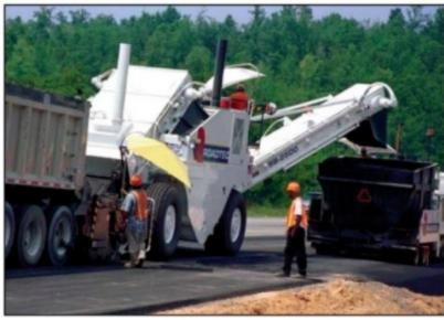
The SB-2500D Shuttle Buggy® material transfer vehicle can store hot mix asphalt and transfer it from a truck to a paver for continuous paving. A patented antisegregation auger remixes materials just before they are delivered to the asphalt paver. The 25-ton (22.7 MT) surge capacity of the SB-2500D allows trucks to unload material immediately and return to the asphalt plant. Options include a windrow pickup head and road widener attachment.
